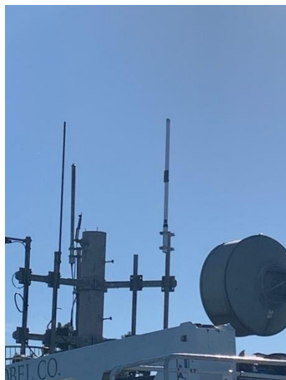
Radio antenna work at the Pt Reyes Site.
