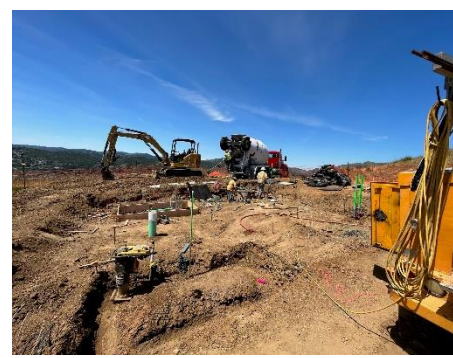
Construction at Skyview
