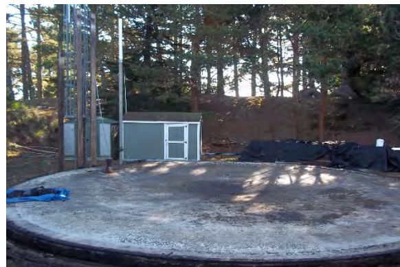
4. Muir Beach Removed Water Tank
