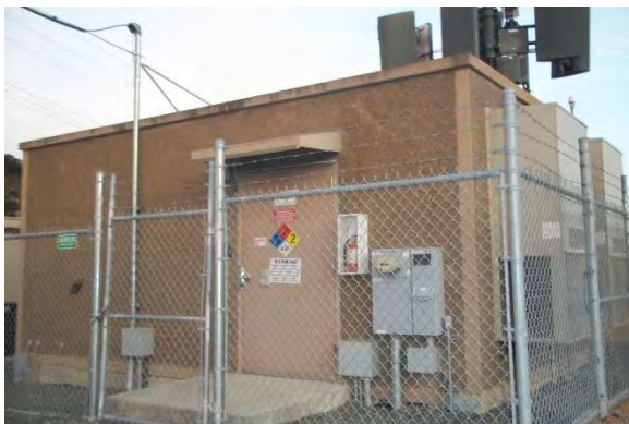
3. Redwood Landfill Communications Shelter
