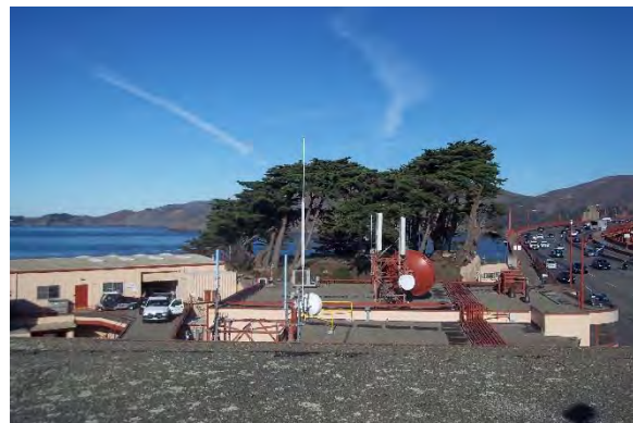
4. Golden Gate Bridge Rooftop Structures
