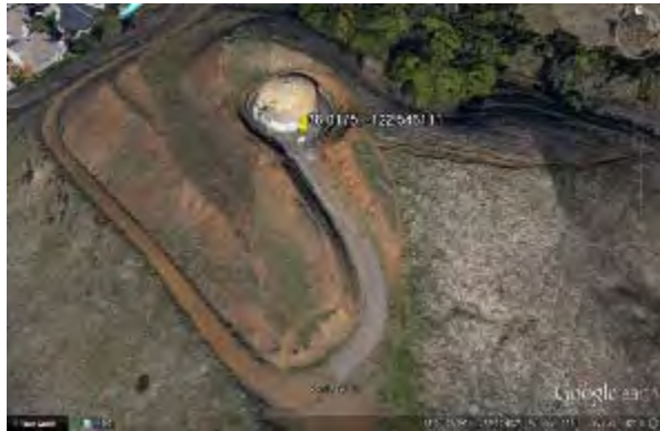
1. EOF Water Tank Aerial View Facing North
