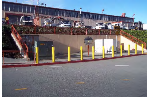
2. Golden Gate Bridge Available Cabinet Space
