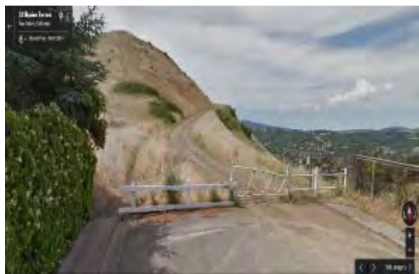
4. EOF Water Tank View From Locked Gate
