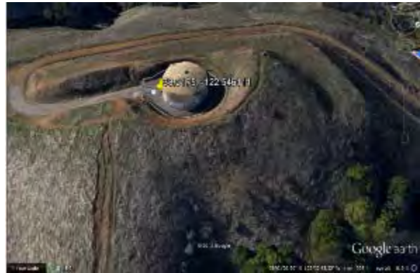
2. EOF Water Tank Aerial View Facing West
