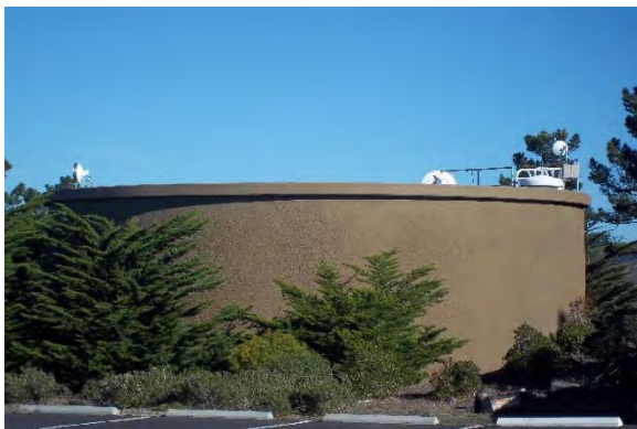
3. Muir Beach Water Tank Facing North
