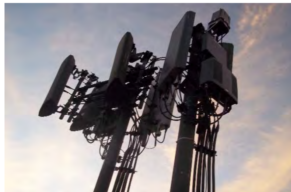
6. Redwood Landfill Tower Structures
